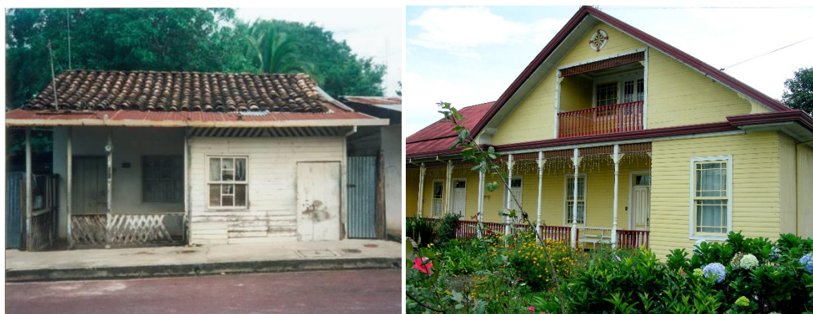
Figure 2-5: Further classification of structures using roof weight and wall condition variables to differentiate expected ductility levels. Left: low expected ductility wooden structure due to heavy roof and bad condition of LLRS. Right: high expected ductility wooden structure due to light roof and good condition of LLRS. Photo sources: http://goo.gl/9uJJLu and http://goo.gl/9uJJLu .
