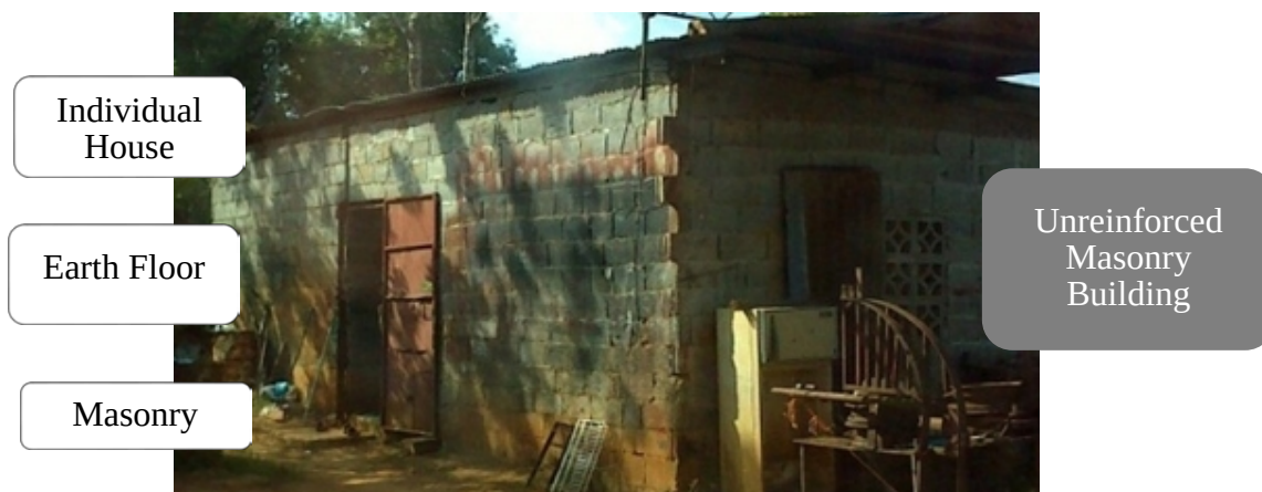
Figure 2-2: Unreinforced masonry structure, identified using three census variables. Photograph source: http://goo.gl/dKTdx0 .
